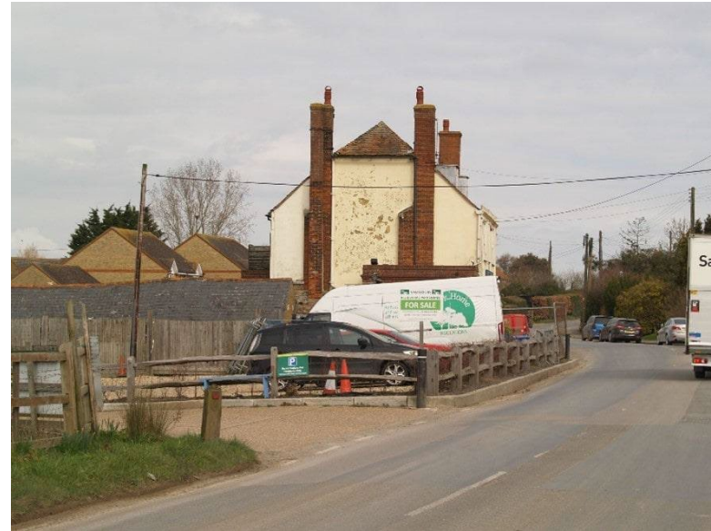
Looking north from Head Hill Road.
