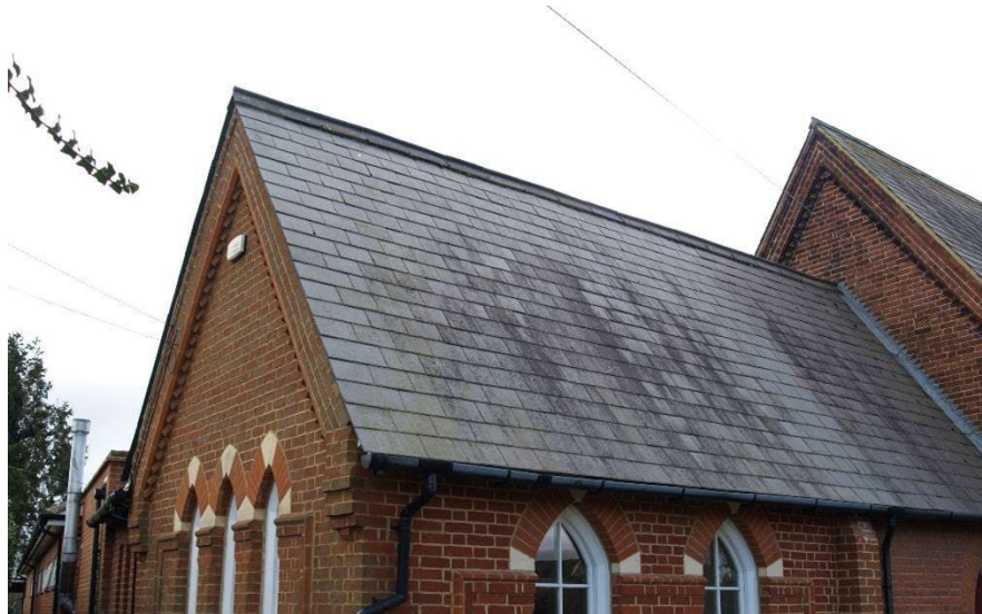
Slate tiles at Graveney Primary School.
