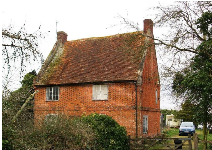
Brickwork to front of Murton's Farm.
