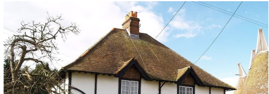
Tiles on roof of Poplar Hall Cottage.
