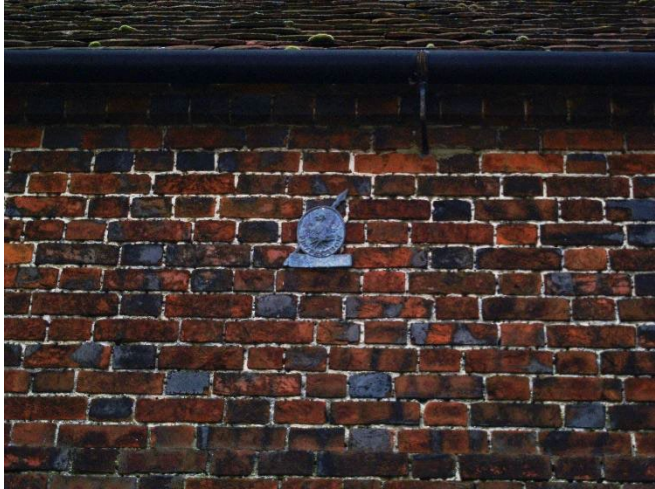
Brickwork on Bridge House.
