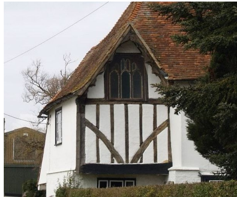
Timber frame visible on Goodnestone Court.
