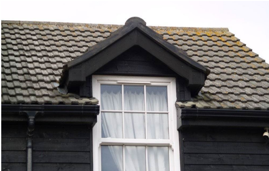
View of the concrete roof tiles used on the Bridge Cottages.
